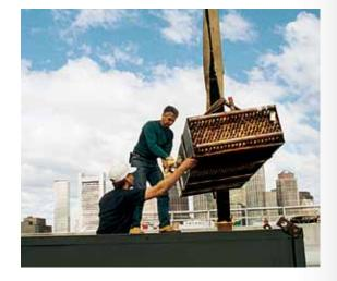
Technicians lower one of 16 made-to-fit replacement coils constructed by Heatcraft for **Boston's World Trace Center**. Since the center's main hall is booked all-year round for conventions, trade shows and special events, the coils had to be scheduled for delivery on Friday so that installation could be done when the convention center was empty.
